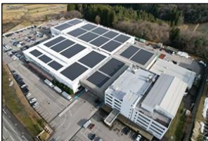
Solar power generation equipments (rooftop)
